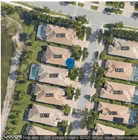
Removal and Grind
