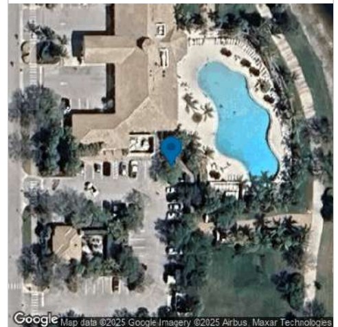
Removal and Grind
