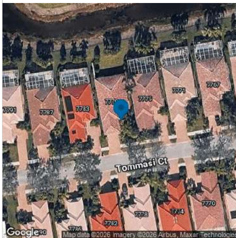
Removal and Grind
